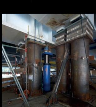
**605 tons locknut cylinders**
